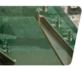
Seismic fittings in the **Planar<sup>™</sup>** | SentryGlas<sup>®</sup> Plus System installation: Alvarado Medical Centre, California
