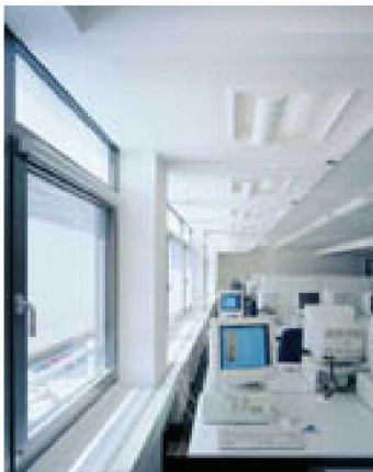
SGG LUMITOP installed in high-level glazing
